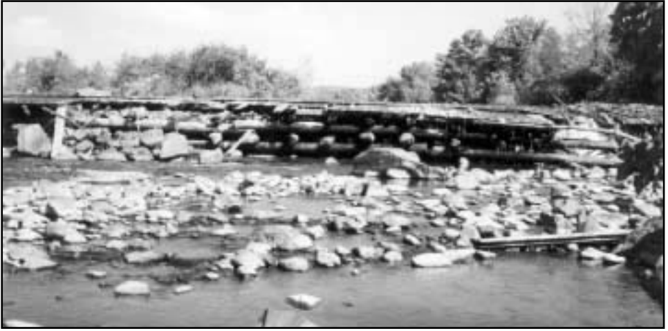
Anaconda Dam ■ Naugatuck River, Connecticut, USA
