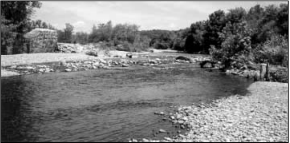
Anaconda Dam ■ Naugatuck River, Connecticut, USA
